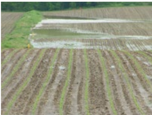
A field terrace intercepts runoff and directs it into a subsurface drainage system.
