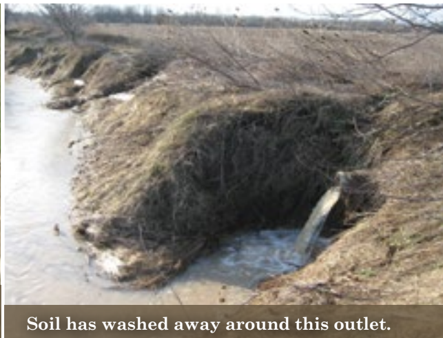
Water flowing across the field has concentrated and broken through the bank.
