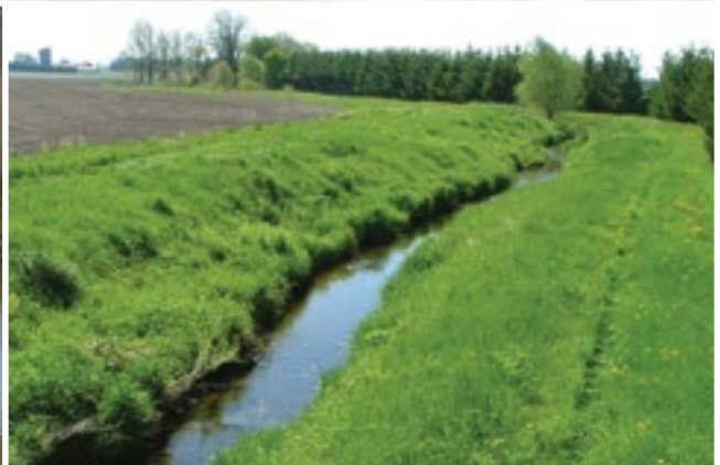
A stone lining with filter-cloth underlay can solve minor erosion problems.
