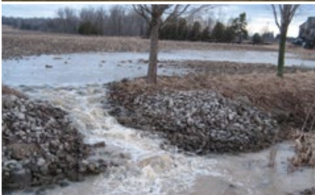
To be effective, a rock-lined spillway is adequately sized, and made of filter-cloth underlay and properly sized angular stone.
