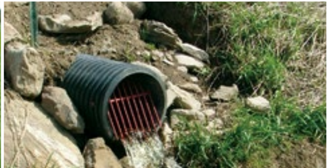
Subsurface drainage outlet pipes should point downstream. They should be protected by a rigid pipe with hinged rodent gate, and rock-lined splash pad with filter-cloth underlay.
