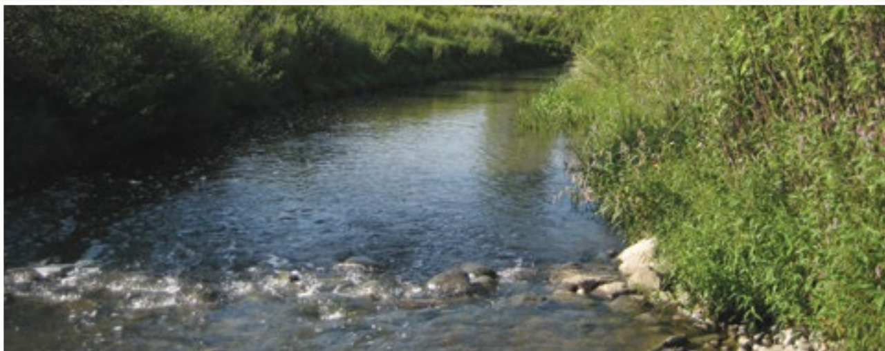
Riffle and pool in drainage channel
