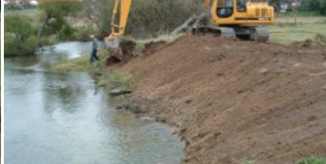
Shaping the bank to accommodate stone
