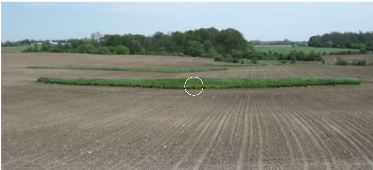
Ground view of WASCoB's riser pipe (circled)
