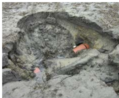
Drainpipe blowout.
