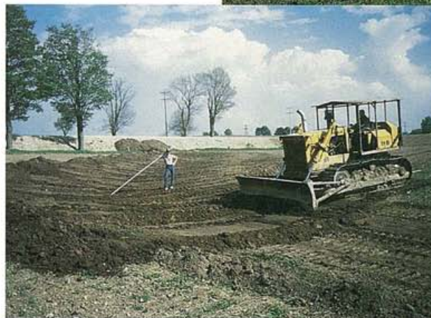
Generally, bulldozers are used to construct grass waterways in Ontario. Proper design ensures a good investment.
