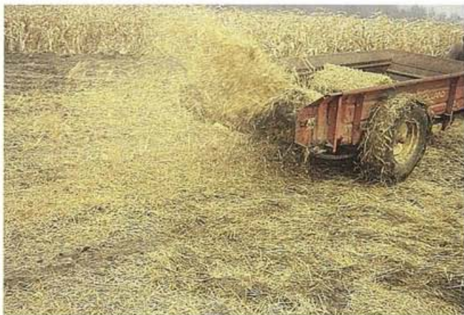
A good dense mat of grass must be established quickly. Straw mulch will help seeds germinate and offer protection against runoff until the grass grows.
