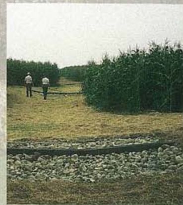
A combination rock and timber control structure reduces the grade and helps control surface flow.
