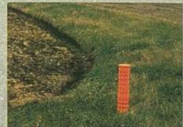
Properly-designed and installed inlets make tile outlet terraces successful. They must be kept clear of debris for efficient operation.
