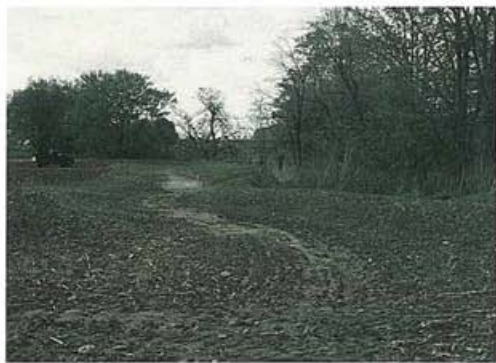
A diversion along a stream directs field run-off to a temporary ponding area. Water then is released slowly into the stream through a vertical pipe inlet leading to a tile drain.
