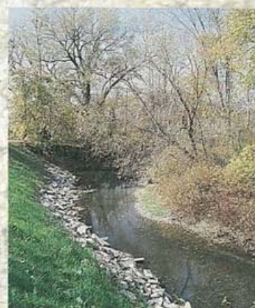
Properly-sized, irregular-shaped rocks with a filter blanket underneath, protect the lower bank while vegetation protects the upper portion.
