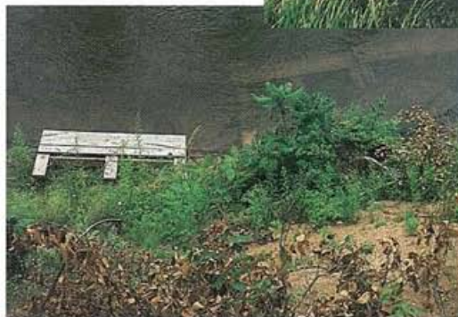
Fish habitat and protection devices, such as "lunker" structures, can also help stabilize banks.
