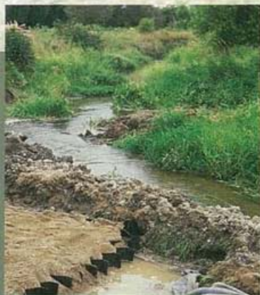
A diversion restricts water flow to one side of this stream while a machinery crossing is installed.
