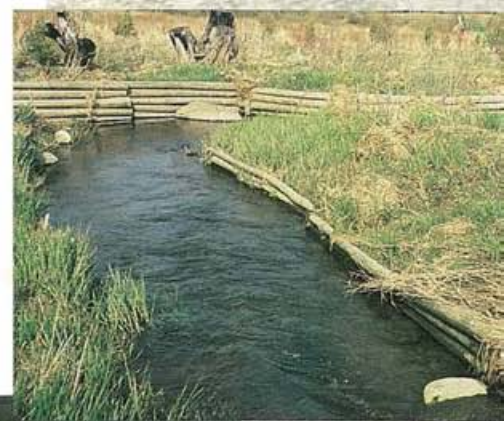
▲ A log crib structure provides bank protection and fish habitat.
