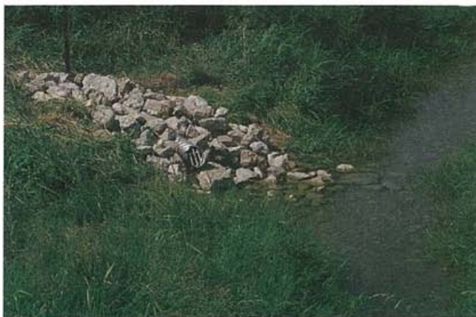
A properly-installed tile outlet.
