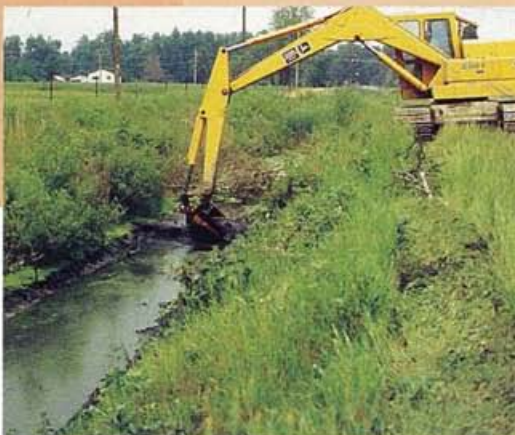
A bottom cleanout removes sediments only. The banks remain untouched and stable.
