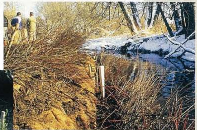
This bioengineering technique involves the placement of bundles of shrub willow or dogwood in trenches along eroding banks. Over time, the banks will look completely natural.
