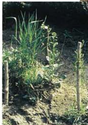
Here, live staking is done with willow whips.
