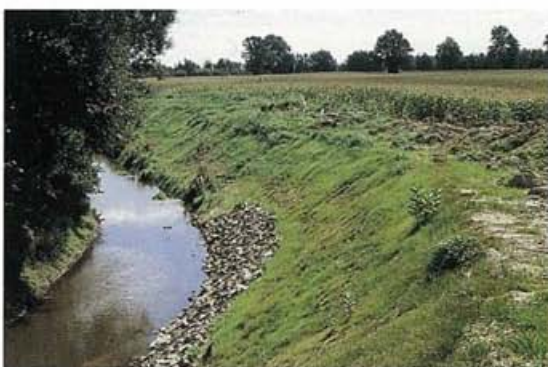
Minimize disturbance by cleaning drains from one side only. In the drain shown here, rip-rap has been added to the outside bend to reduce erosion.
