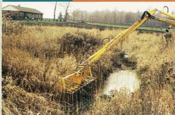
Excessive vegetation in the channel can be removed to allow more efficient flow. In some cases, this will even improve habitat value.
