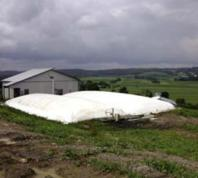
Using anaerobic digestion technology, liquid manure can be processed to generate biogas for energy and to reduce methane emissions.
