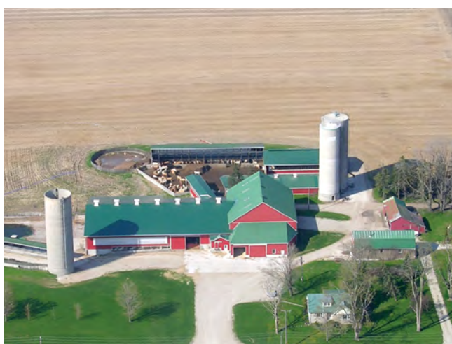
Relining silo walls helps to seal in seepage and maintain structural integrity.
