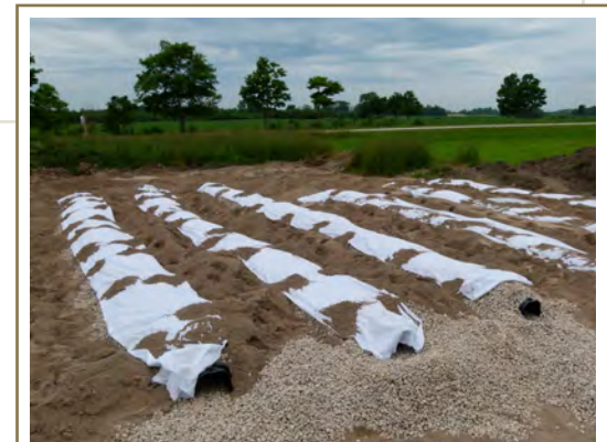
This treatment trench area will be fenced off from livestock and vehicles once installation is complete.
