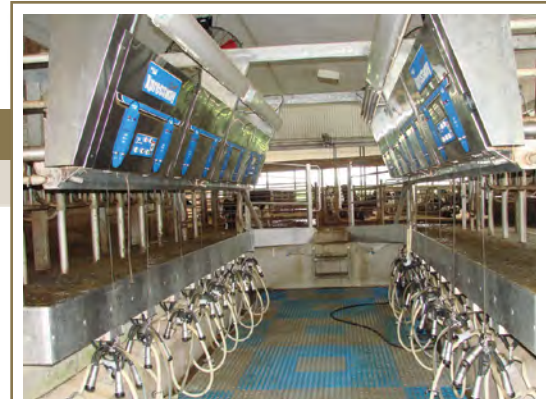
Before washing the milking centre floor, clear the solids away with a shovel and broom.
