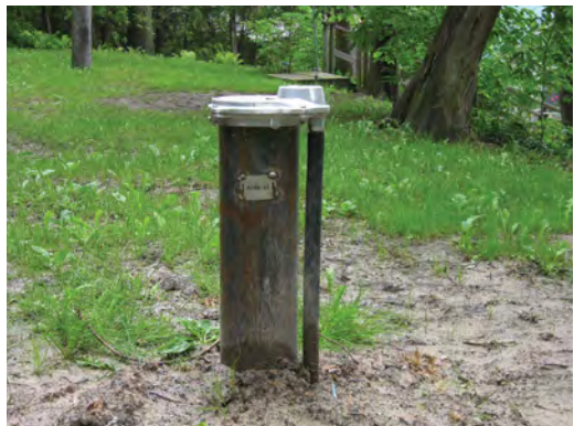
Regrade soil around the well to prevent surface water from ponding near the casing.
