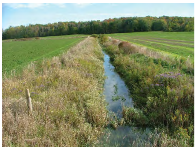
A thick cover of vegetation will stabilize the banks and greatly reduce maintenance requirements.
