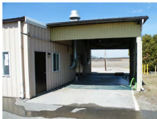
A dedicated mixing/loading area will reduce the risk of surface or ground water contamination.
