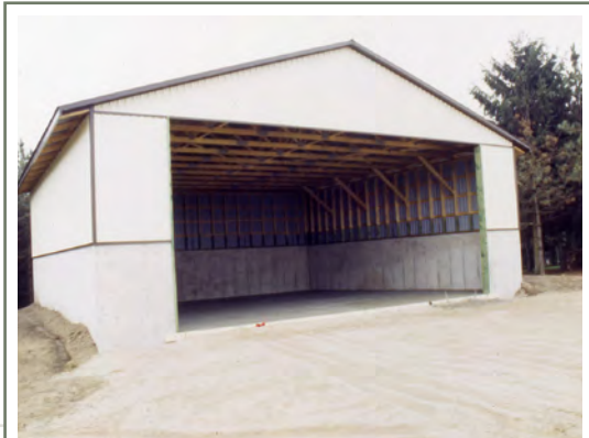
A permanent roof is the best way to keep rainwater out of the mixing/loading area.
