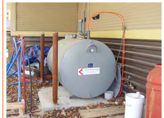
Lines are often the source of leaks.
