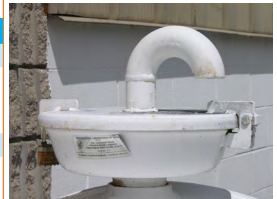
The overfill device is designed to prevent filling to more than 95% capacity.
