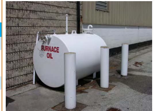
Confirm fuel oil storage is ULC-approved.
