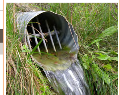
Drainage tiles are a conduit to surface water, and composting sites should be located at least 10 m (33 ft) away.
