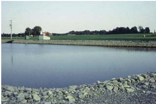
Dugout ponds work best in poorly drained sandy soils when they can be replenished by ground water.
