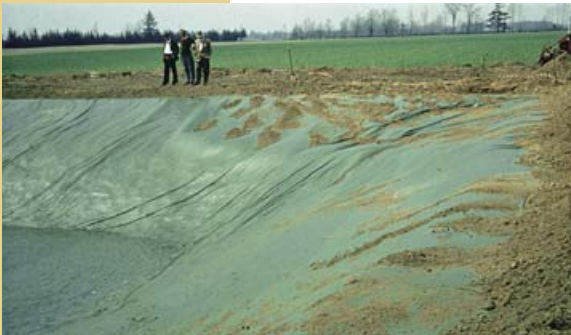
Dugout ponds in drier medium-textured soils and drier coarse-textured soils may require artificial liners to reduce water loss.
