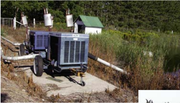
This diesel-powered pump on a pad is drawing water from a pond.
