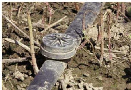
This is a drip emitter, which provides a point source for water discharge.
