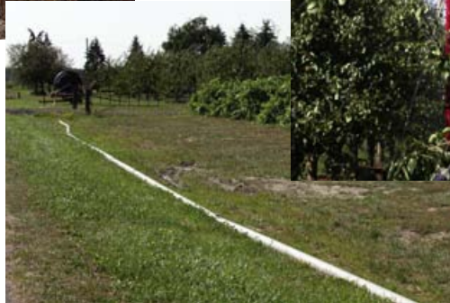
A conduit pipe carries water to the field.
