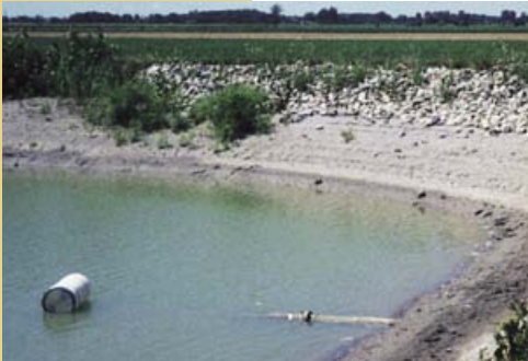
This large reservoir stores water for the growing season. It is filled with water pumped from drainage ditches during the winter and spring, and is gradually emptied over summer months.
