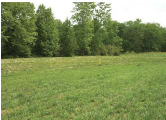
This is a well-constructed WaSCoB with established forage cover.
