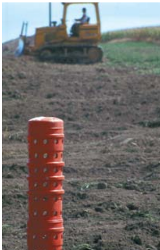
WaSCoBs are earthen embankments across draws, with retention basins and drop pipe structures to convey water to an adequate tile outlet. The duration of temporary ponding is carefully engineered to reduce the risk of damaging the crop.
