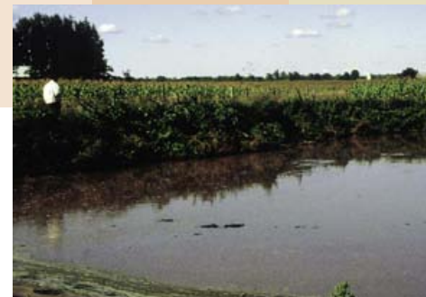
Earthen storages – with proper siting, site characterization and design – can be effective storages for liquid manure, runoff and washwaters.
