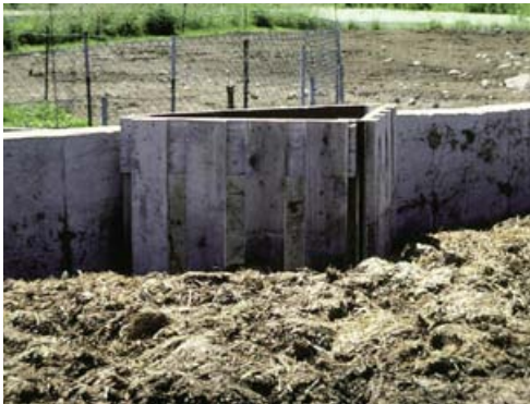
A solid storage with a separate runoff system will contain all liquids – but will require two means of application.
