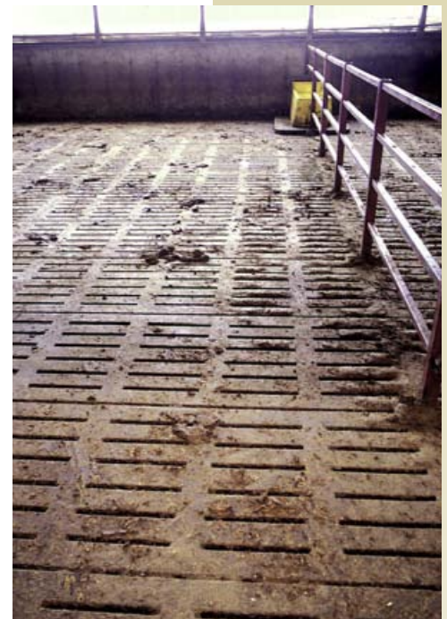
Manure is transferred to an in-barn storage by the action of animals' hooves.
