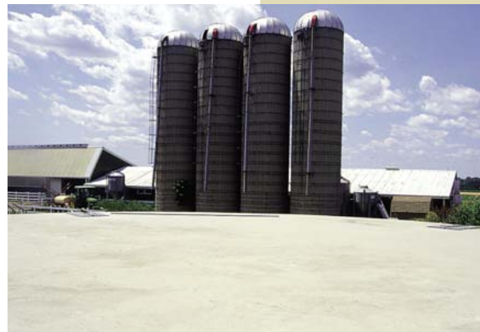
Floating covers can be effective alternatives for circular storages.
