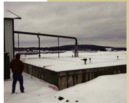
Covered liquid manure storages emit fewer odours.
