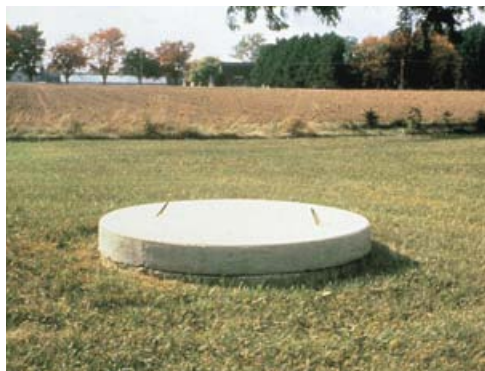
Manure should not be applied within 30 metres (100 ft) of private large-diameter wells.
