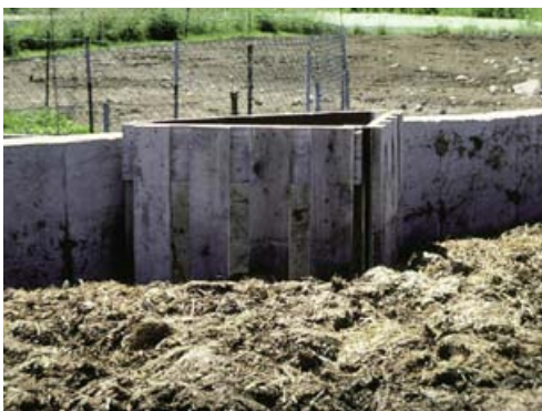
A solid storage with a separate runoff system will contain all liquids – but will require two means of application.
