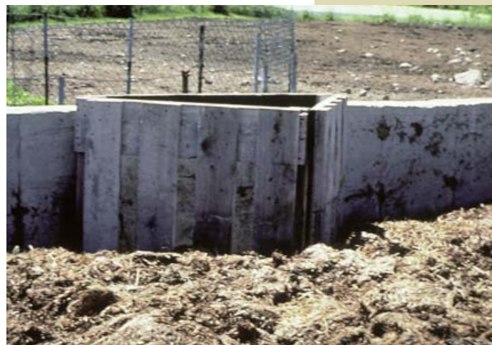
Solid manure systems with separate liquid runoff storages can handle large volumes of bedding and liquids.
