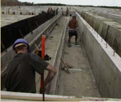
Raceway systems consist of two or more interconnected channels that lead back to one circulation or agitation point.
