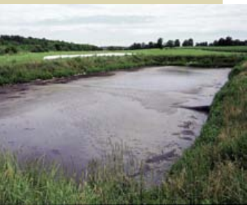
Although less expensive than concrete storage, open earthen storages require a thorough site investigation and may require liners to protect groundwater from contamination.
