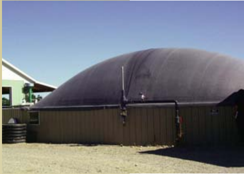
The biogas produced by anaerobic digestion units can be burned for heat or used to generate electricity.
