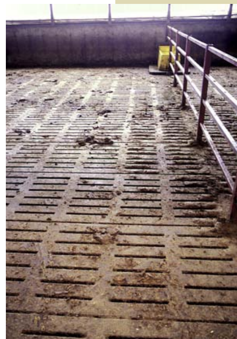
Manure is transferred to an in-barn storage by the action of animals' hooves.
