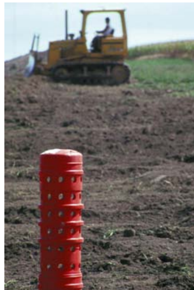
Erosion control structures, such as Water and Sediment Control Basins (WASCoBs), will help reduce sediment load from cropland runoff.
