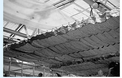
A double polyethylene-covered greenhouse reduces air infiltration losses. But unless it has an infrared-treated film, infrared radiation can be transmitted out of the greenhouse.
