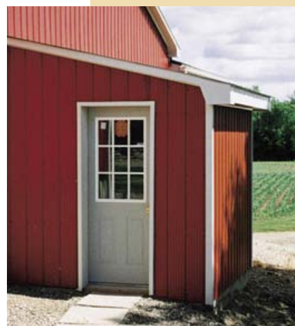
Built-on storages require ventilation to the outside, an outdoor entrance, and proper firewalls.
