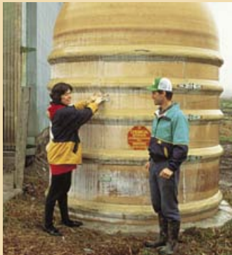
One end of a used fibreglass fuel tank was attached to a seamless concrete floor (with 150 mm [6 in.] curb) to create this unique pesticide storage. Total material cost was $185.
