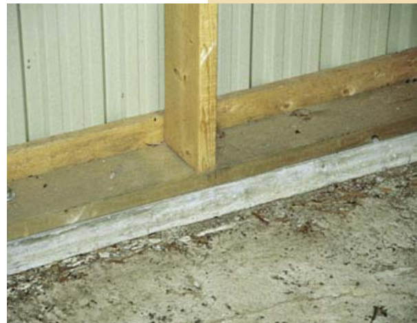
The base plate needs to be secured to the poured floor curb with anchor bolts.
