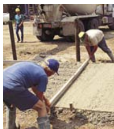
Step 3 Use float to finish poured floor.
