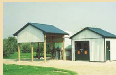
Pesticide storages should be located to minimize risk of contamination of groundwater, surface water, natural habitats, livestock feeds, and human activity.
