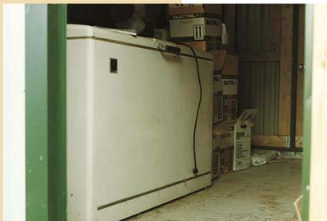
A well-insulated frost-free cabinet located inside a pesticide storage can be heated with two low-wattage light bulbs.
