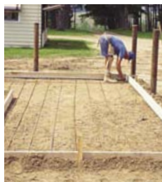
Step 2 Build forms.
