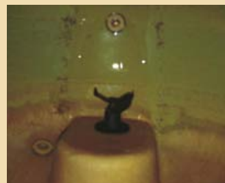
Check agitator paddles and shafts for breakage and wear.
