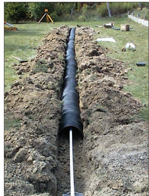
Single line shallow buried trench.
