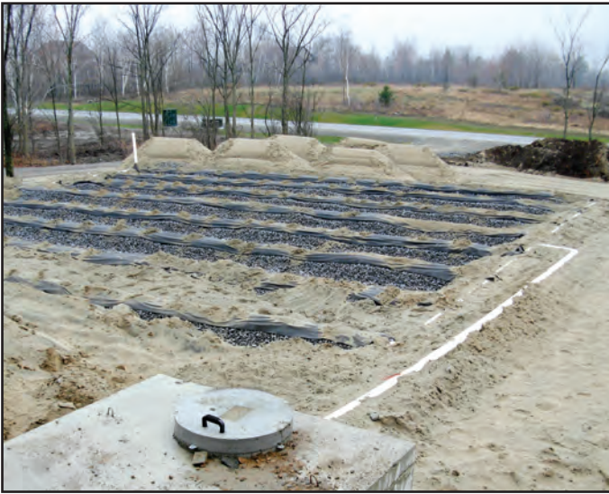
Leaching bed with perforated PVC drain pipes.
