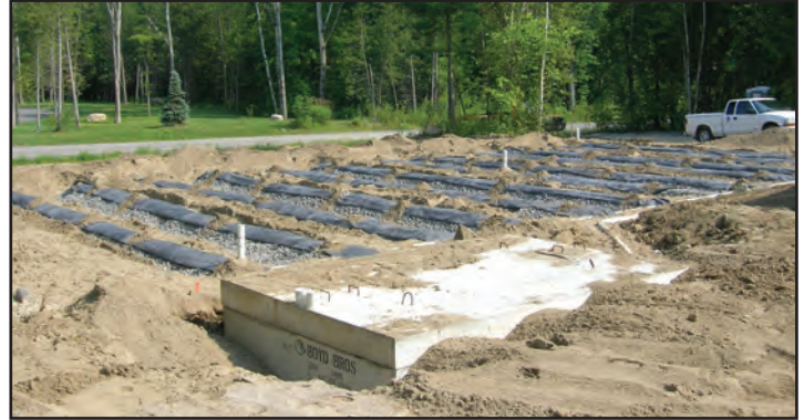
Septic tank and leaching bed.
