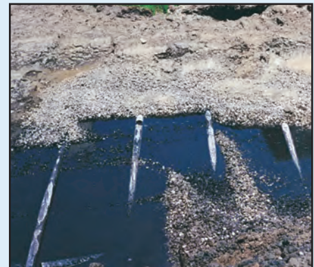
A failed system exposed.
