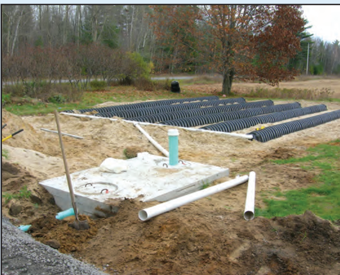
Leaching bed with gravelless trench technology.
