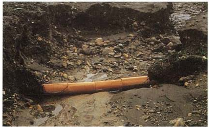
Gully erosion refers to a rill that is too large to be crossed with equipment and cannot be filled in by tillage.
