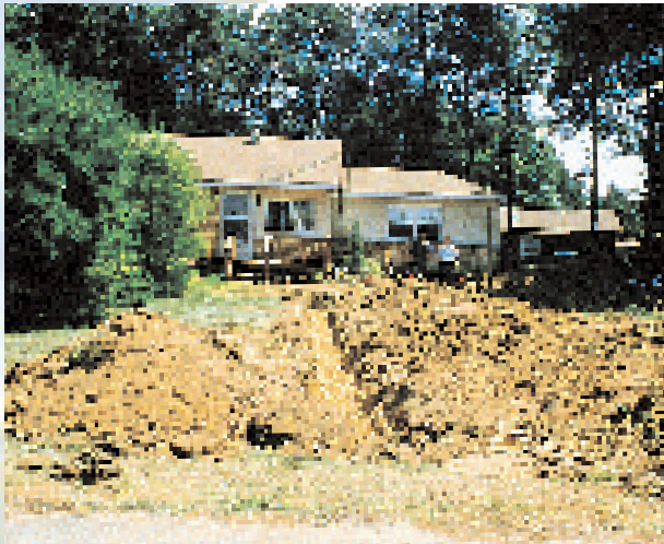
Treatment trench leaching bed installation.
