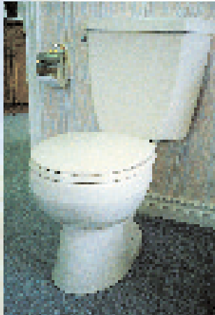
Low-flush toilets and toilets with dams and displacement bags will use less water.
