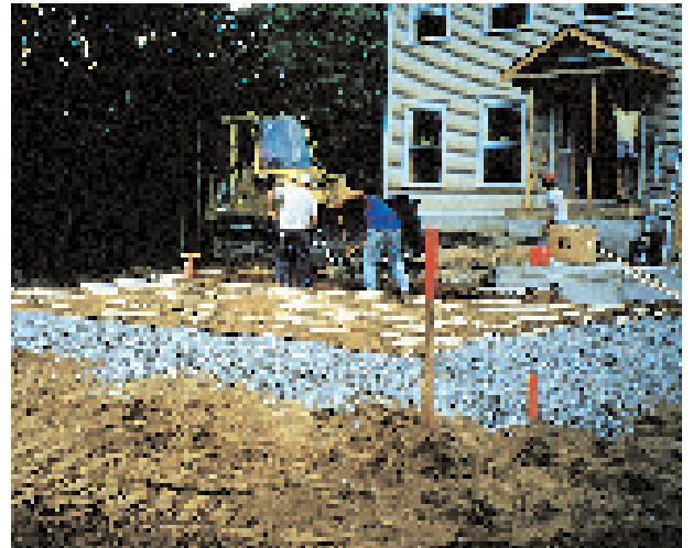
Raised beds are installed over shallow bedrock in many areas in Eastern, Northern, and Central Ontario as well as in areas with heavy clay soils.
