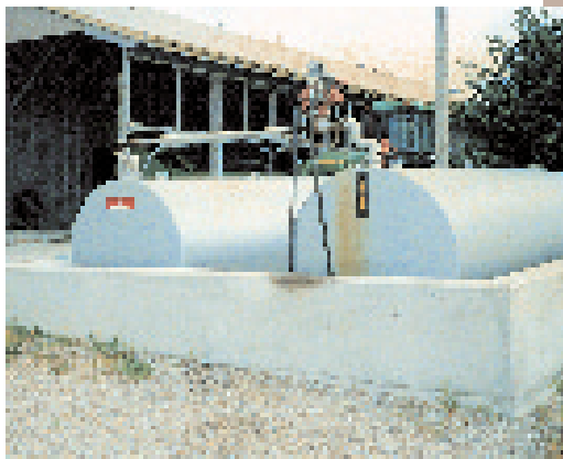
An above-ground fuel tank should be diked and sized to contain 110% of its volume.
