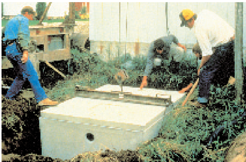
Many dairy farmers have installed a treatment/disposal system to prevent milkhouse washwater from directly polluting streams.
