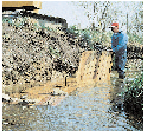
Installing lunker structures along a municipal drain.
