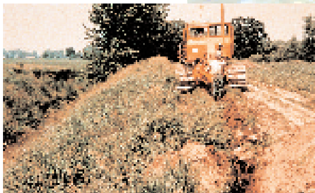
Ground water seepage can cause slumping of streambanks. To control slumping, install tile drains along a drain bank.
