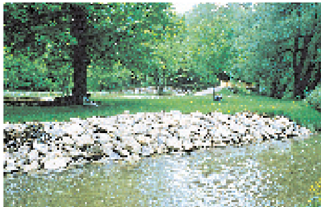
Rock can protect pond banks from erosion and damage from burrowing animals.
