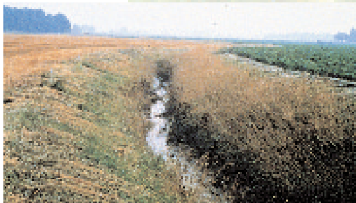
A well-constructed and maintained open ditch. Grass buffers are left to provide stability to the drain bank and filter out soil moving in runoff.
