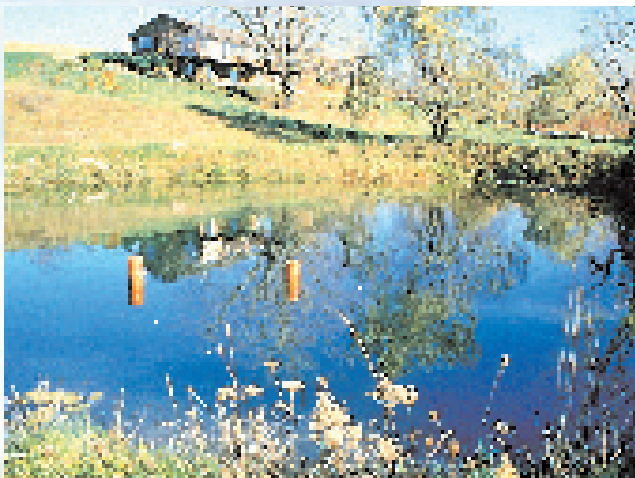
Vertical intake pipes are used to adjust water levels in this embankment pond constructed across a natural drainageway.
