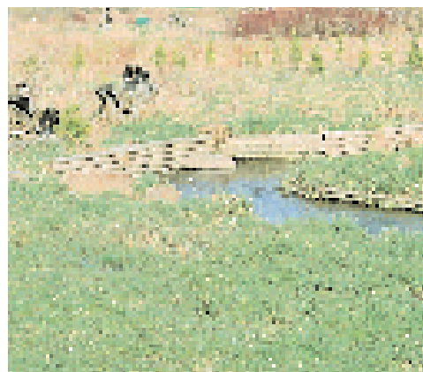
Before restoration, this channel flows wide and shallow, offering little opportunity for aquatic life. Following the reshaping of the channel to a natural flow path, the water is deeper and moves faster to provide better flow characteristics and fish habitat.
