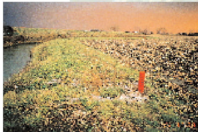
In this drop inlet system, a diversion constructed along a drain intercepts surface water and directs it to a single drop pipe inlet.
