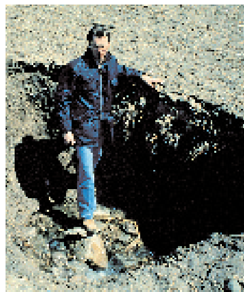
A tile blowout or wash-in indicates immediate attention is needed to repair the tile drain.
