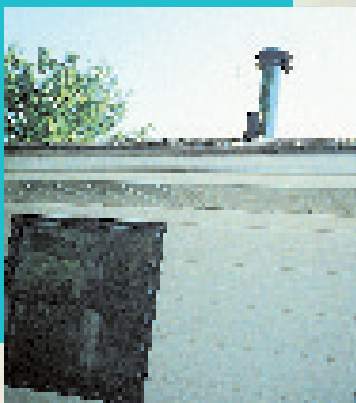
The septic tank will generally be located in line with the main roof vent on your house.
