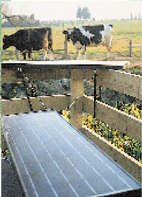
A solar-powered watering system: photovoltaic panels use the sun to charge batteries, which in turn power a pump that distributes water to meet livestock needs.
