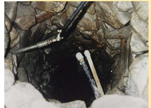
Shown here is a drilled well inside an old dug well. Surface water and shallow groundwater can collect in the old well and drain into the new one, causing contamination problems.
