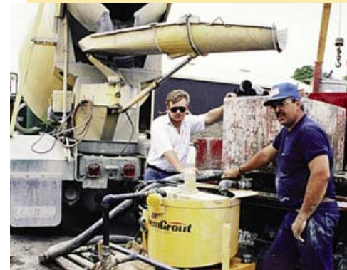
Contractors grout the annular space around the outside of the casing of a newly constructed well.
