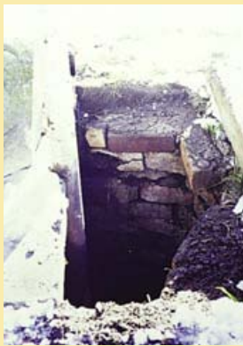
With or without a proper cover, the brick lining on this old well can present problems.
