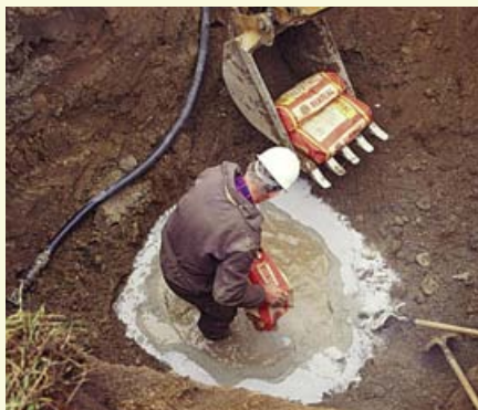
A final plug of bentonite was created to prevent any movement of liquid down the old casing.
