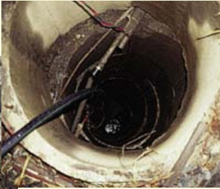
Prior condition: old dug well had been replaced with a drilled well nearby, and old well presented a risk to groundwater quality and personal safety.
