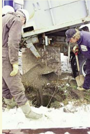
Licensed contractors were hired to plug the well. Pea gravel was added to the well to provide a solid base over some rock and other debris that had been pitched into the well over the years. In some cases, debris removal would be required.
