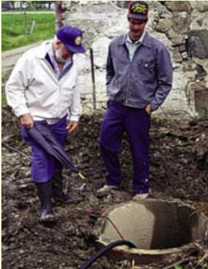
Bentonite clay was added to form a plug at the water-bearing layer.
