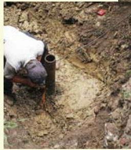
Steel casing was trimmed down and an adapter plate welded on to accept casing extension.
