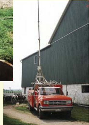
A submersible pump was removed from well.
