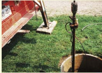
A submersible pump was removed from well.
