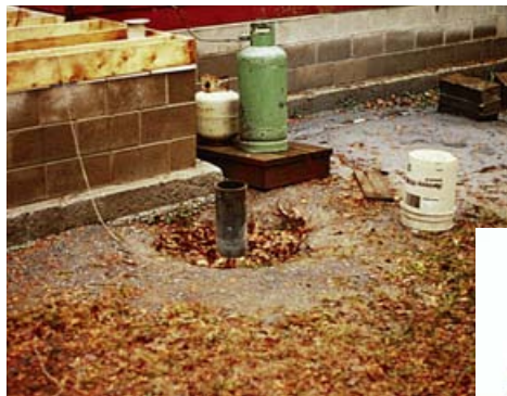
This is a problem situation: there is no watertight cap, and settling around the casing suggests a poor annular seal.
