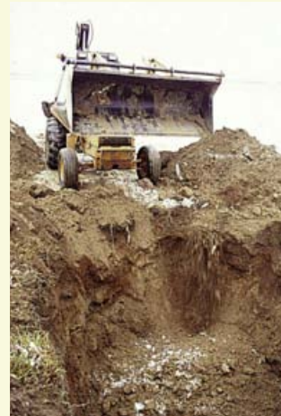
The hole was filled with clean clay soil, mounded to direct surface flows away, and seeded. A Water Well Record describing the procedure was completed and filed with the authorities. Total material and labour costs were $695.*
