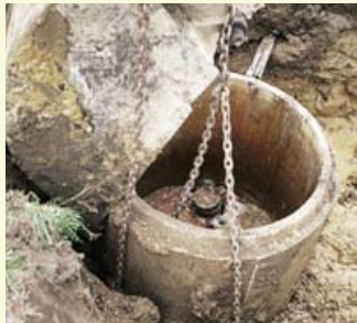
A backhoe removed well tile that served as the pit, and opened up hole around steel casing.
