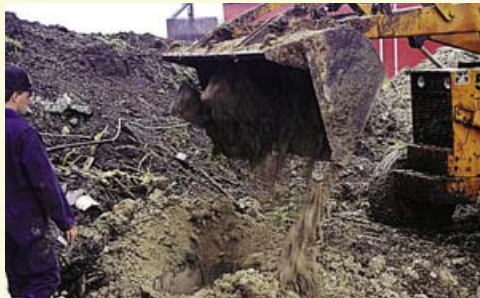
Clean clay fill was added to within 3 metres (10 ft.) of the ground surface.
