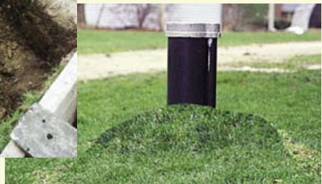
Hole was backfilled and mounded to direct all surface flows away. Electrical service was hooked up, and a tight-fitting vented cap secured. Total cost of materials and labour provided by a licensed well contractor was approximately $900. (The scope and cost of each job will of course vary. Always get an estimate.)
