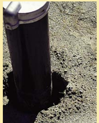
If not sealed, the annular space around this drilled casing could convey contaminated surface water directly into the aquifer.
