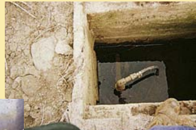
The well cap is submerged in this pit. A faulty seal could lead to contamination of the well.
