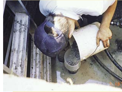
Pouring dry bentonite down an unused drilled well casing may not form an effective plug. The material can stick or form a bridge in the casing, leaving gaps in the seal.
