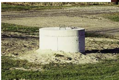
Using clean clay, mound the ground around the outside of the well casing.
