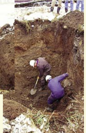
The upper concrete well tiles were removed to expose the clay soil fill.
