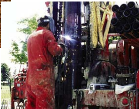
Joints between sections of steel casing are welded as they are lowered into the well.
