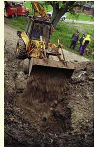
Hole was filled in with clay soil, mounded to direct away surface flows, and seeded. Total cost for materials and labour provided by a licensed contractor was approximately $600*. A Water Well Record describing the procedure was then filed with the proper authorities.
