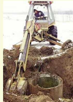
The upper concrete well tiles were removed to expose the clay soil fill.
