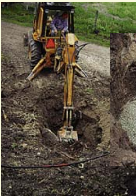
Top few concrete well tiles were removed. A second plug of bentonite was placed over the remaining tiles to prevent any downward movement of liquids into the old well.
