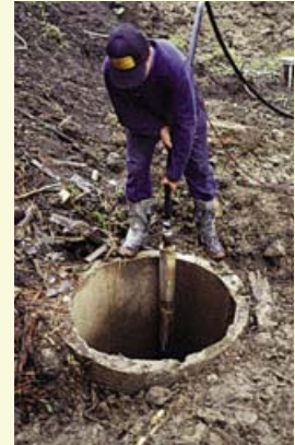
Standing water was removed with a submersible pump.
