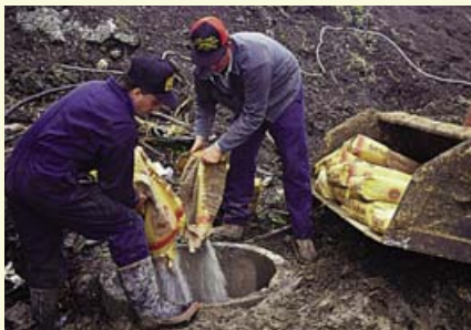
Bentonite clay was added to form a plug at the water-bearing layer.
