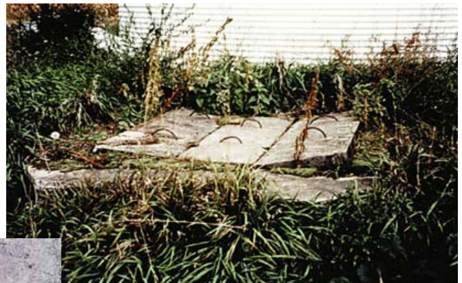
These poorly maintained wells will not prevent surface water from entering. Water samples from these wells would have high counts for Total Coliform and possibly high counts for E. coli .
