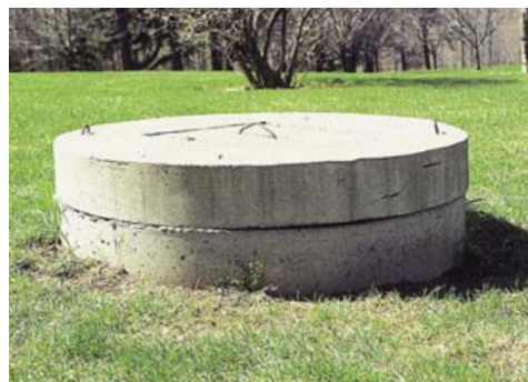
Large-diameter wells typically use concrete casing. Older installations may have been cased with brick, stone, timber or corrugated steel.
