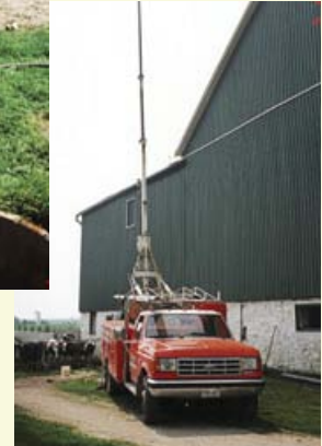
A submersible pump was removed from well.
