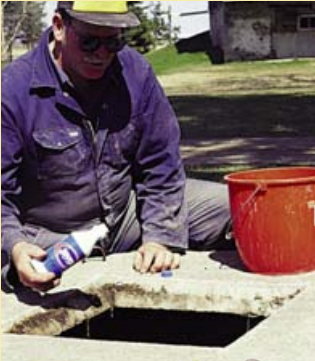
Liquid bleach can be carefully administered to a well to control bacteria problems.
