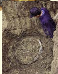
Top few concrete well tiles were removed. A second plug of bentonite was placed over the remaining tiles to prevent any downward movement of liquids into the old well.
