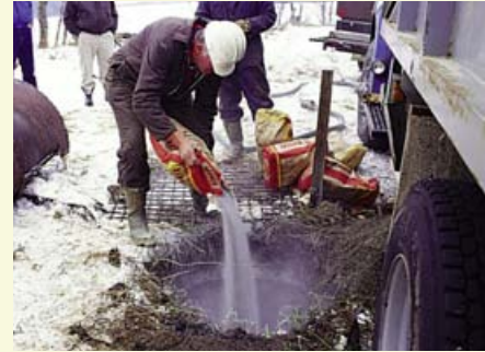
A plug of bentonite clay was formed at the water-bearing layer.
