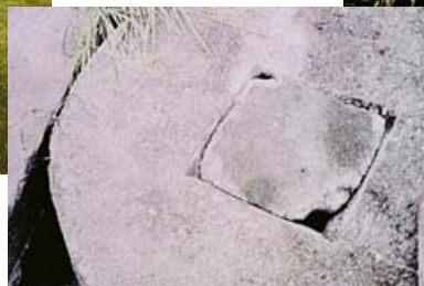
These poorly maintained wells will not prevent surface water from entering. Water samples from these wells would have high counts for Total Coliform and possibly high counts for E. coli .
