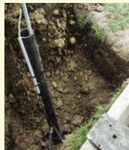
Hole was backfilled and mounded to direct all surface flows away. Electrical service was hooked up, and a tight-fitting vented cap secured. Total cost of materials and labour provided by a licensed well contractor was approximately $900. (The scope and cost of each job will of course vary. Always get an estimate.)
