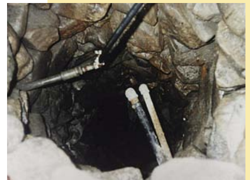
Shown here is a drilled well inside an old dug well. Surface water and shallow groundwater can collect in the old well and drain into the new one, causing contamination problems.
