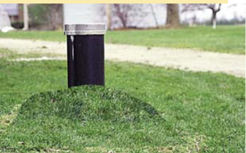
When upgrading an existing well, make sure the well casing extends 0.4 metres (16 in.) above finished ground level.
