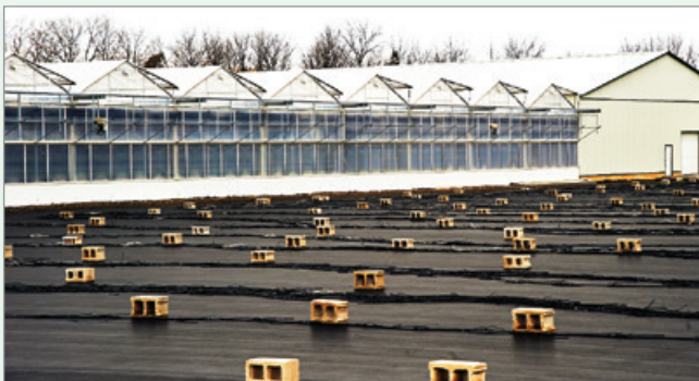
A compacted surface and an impermeable barrier will assist in collecting any nutrient rich water from your outdoor collection area.
