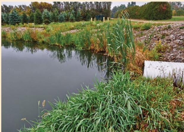
**Nutrient and sediment levels in runoff can be reduced using treatment BMPs such as constructed wetland biofilters with settling ponds as the first step in filtration.**
