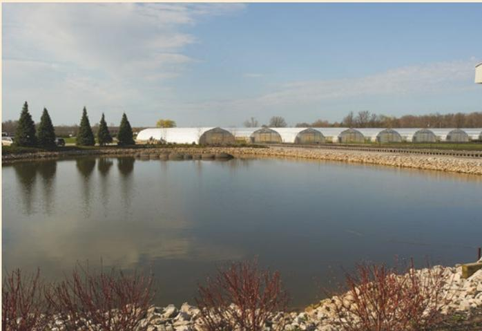
**Irrigation ponds should be sized and constructed to be large enough to meet your design requirements (e.g. irrigation needs, runoff from production area during the growing season).**
