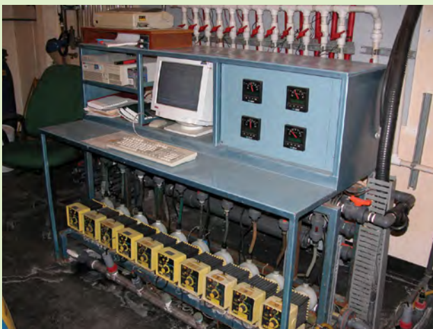
Multi-head injector systems allow managers to match nutrient application to crop needs, according to results of weekly solution analysis.
