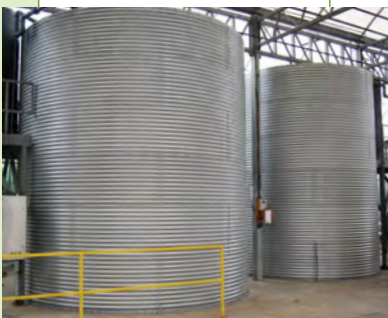
Leached nutrient feedwater is nutrient-rich and should be collected and stored separately from other greenhouse wastewaters.
