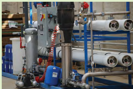
Reverse osmosis will remove salts (nitrates, sulphates, carbonates), pathogens, and other micro-organisms from irrigation water.
