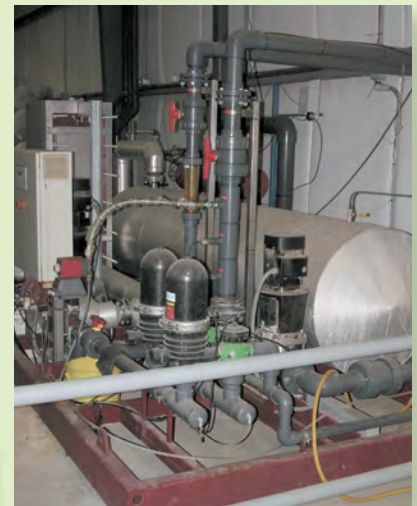
Reverse osmosis will remove salts (nitrates, sulphates, carbonates), pathogens, and other micro-organisms from irrigation water.
