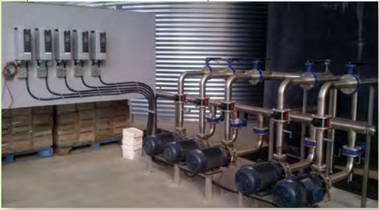
Use of technologies such as variable-speed soft-start irrigation pumps improves precision of irrigation scheduling.
