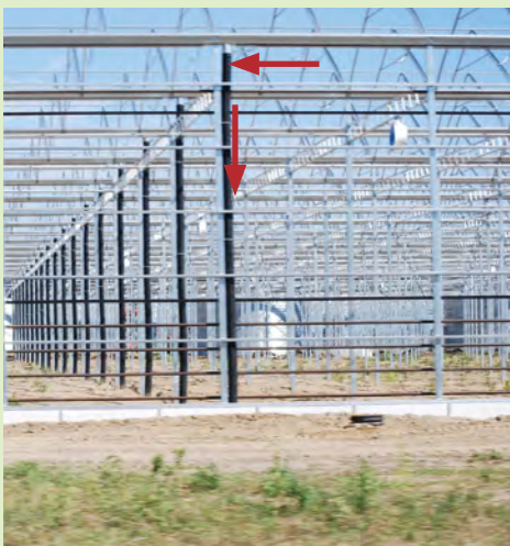
This greenhouse under construction features downspouts to direct rainwater to storm water retention pond.
